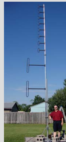
Swing base section out, align, bolt flanges together and erect.
